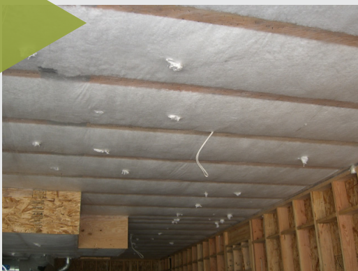
POLAR BLANKET INSULATION IN GARAGE CEILING
