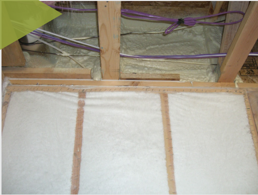
SPRAY FOAM INSULATION IN RIM JOIST
