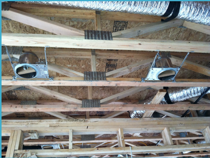
INSTALLING DUCTS INTO OPEN WEB TRUSSES IN FLOOR
